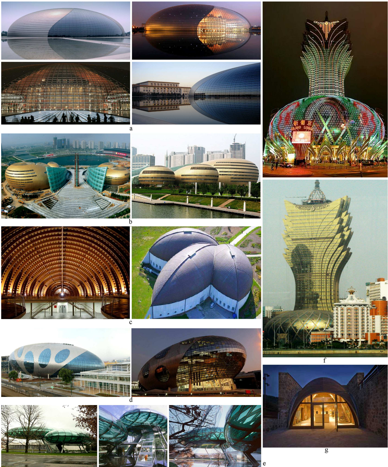
Fig.4. a. The National Centre for the performing Arts “The egg” Built for the Amazing Olympic Architecture in Beijing, China; Fig.4. b. Henan Art centre, China; Fig.4. c. Jurassic museum (MUJA), Asturias, Spain; Fig.4. d. Infosys Company in Pune, India; Fig.4. e. Nardini distillery in Bassano del Grappa, Italy; Fig.4. f. ; Fig.4. g. Saltworks at Añana, Spain.
