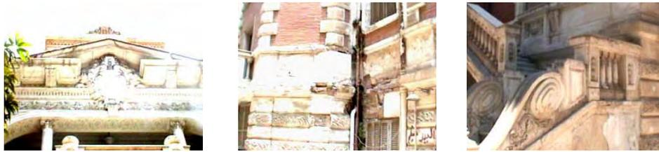
Fig.9 deteriorated parts due to the moisture and atmospheric effect.
