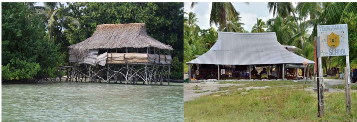
Fig. 3: Left: the roof of a traditional house made with pandanus leaves. Right: example of a galvanized sheet roofing.
