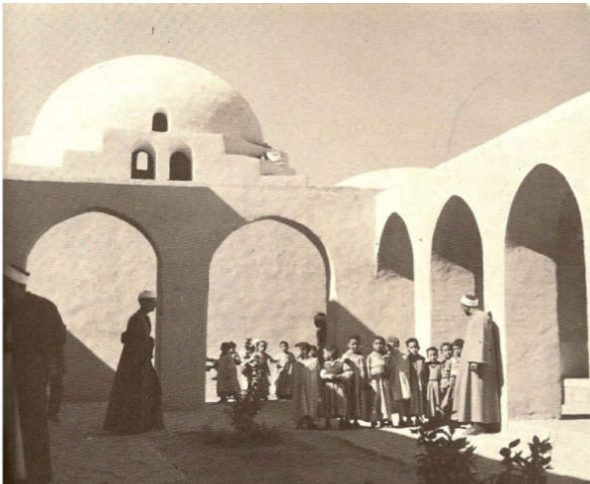
Fig. 3. Viollet R., New Gourna Boys, Primary School (tratto da Taw T., "New Gourna Village, Luxor, Egitto", Architecture-in-Development , 2011).
