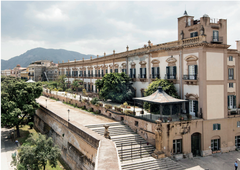
Figure 11 – Palermo Butera palace, waterfront façade (Sandro Scalia).
