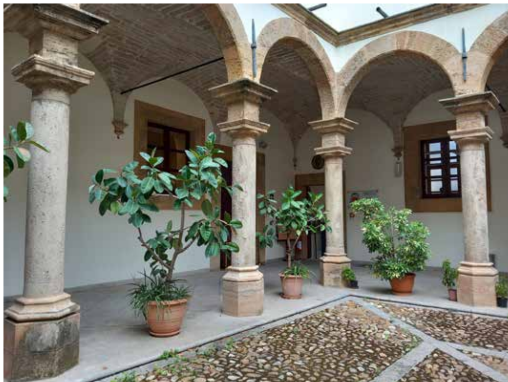
◇ Fig. 7 – Palermo. Archbishop's Seminary, ground-floor loggia with columns possibly made of Santa Maria di Gesù stone (photograph by the author).
