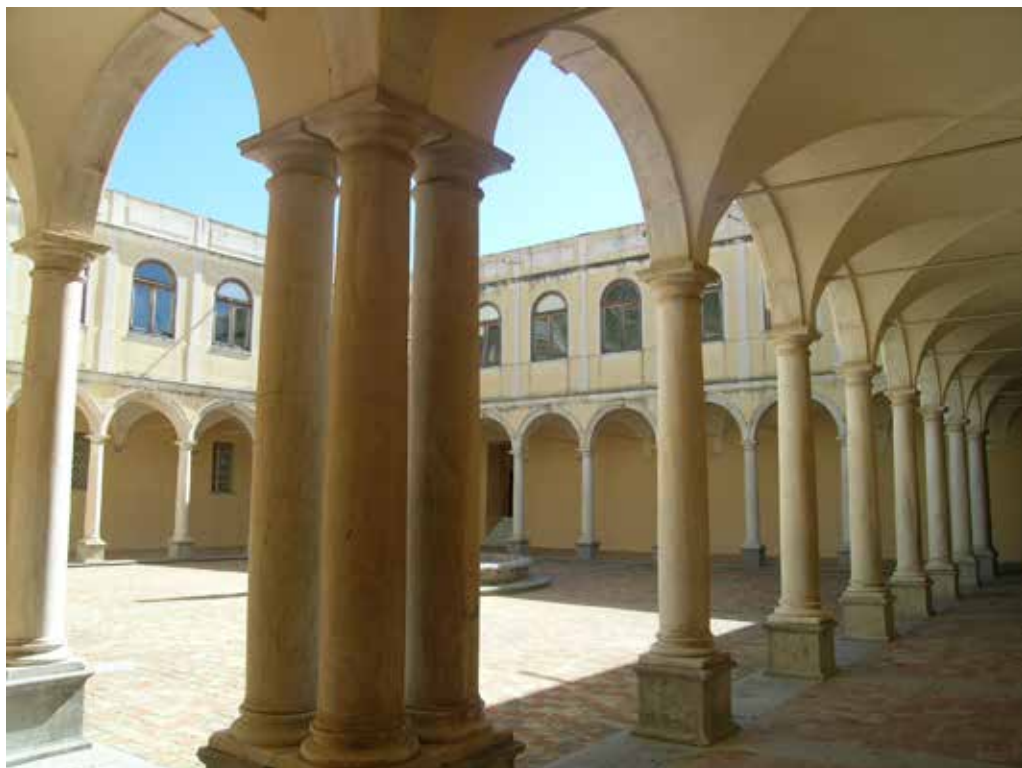
◇ Fig. 3 – San Martino delle Scale (Palermo). Benedictine Convent, cloister, detail of the corner solution with three Carrara marble columns.
