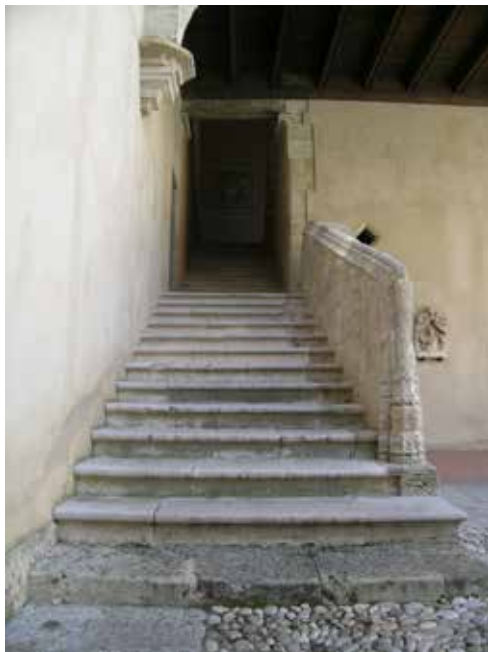
◇ Fig. 9 – Palermo. Palazzo Abatellis, external staircase with steps made of Termini stone (photograph by the author).
