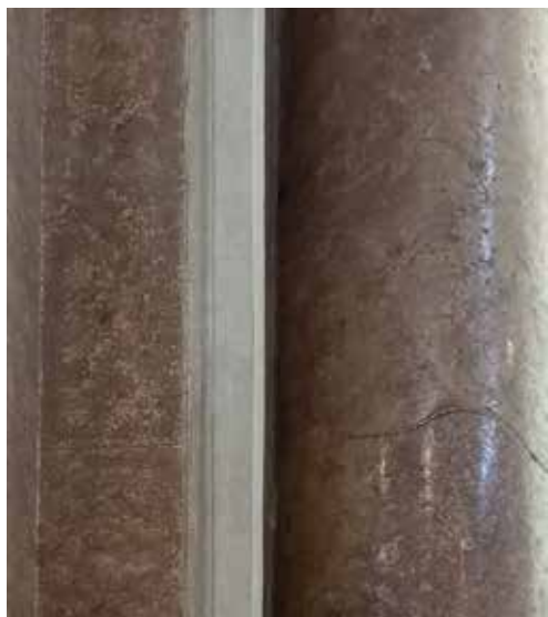
◇ Fig. 4 – Palermo. Church of Sant'Eulalia dei Catalani, interior view, non-monolithic column in Jaspes de Tortosa with a detail of the faux stucco veining following the irregular pattern of the fractures (photograph by the author).
