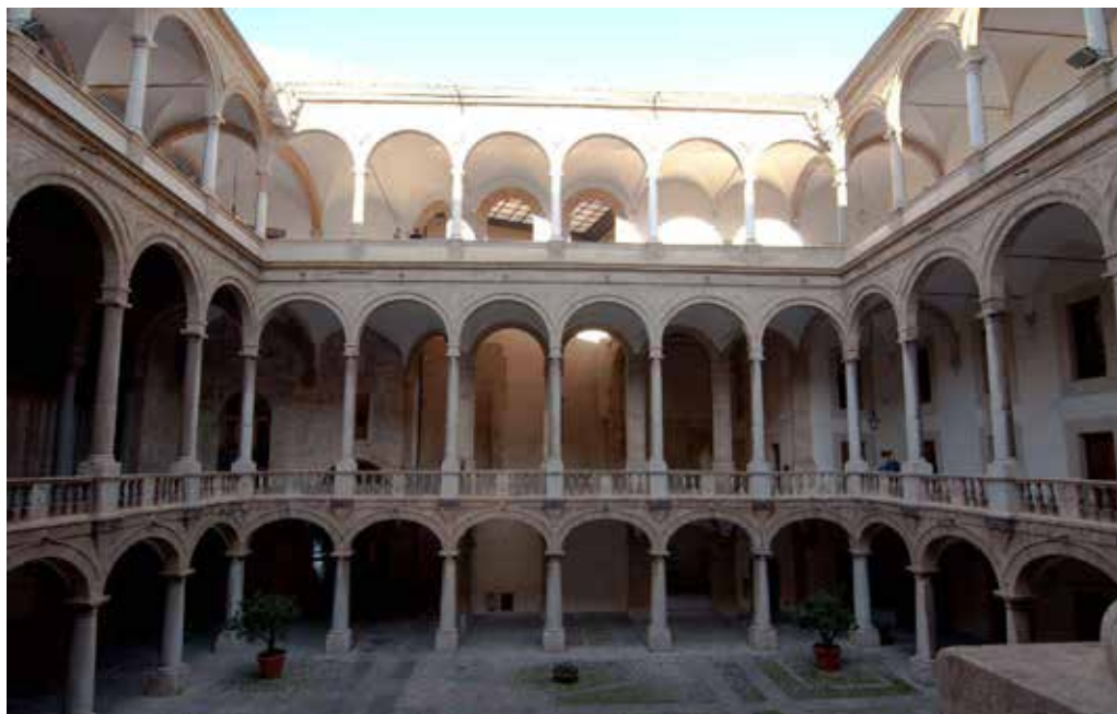
◇ Fig. 15 – Palermo. Royal Palace, Maqueda Courtyard, triple colonnade made of Billiemi stone (ground floor) and Monte Pellegrino stone (first and second floors) (photograph by the author).
