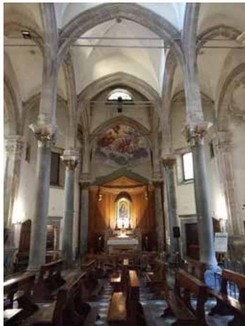
◇ Fig. 1 – Palermo. Church of Santa Maria di Portosalvo, interior view, detail of the tall “sovrassesti” above the Carrara marble column capitals (photograph by the author).
