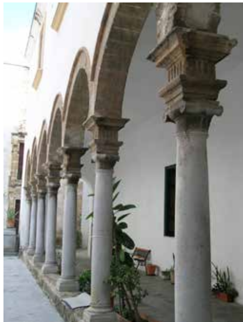
◇ Fig. 12 – Palermo. Convent near the Church of Santa Maria del Carmine, cloister colonnade made of Termini stone (photograph by the author).
