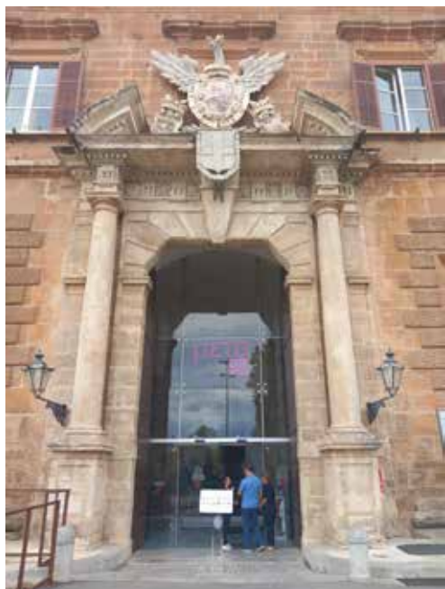
◇ Fig. 8 – Palermo. Royal Palace, external view, Porta del Corpo di Guardia with elements made of Santa Maria di Gesù stone (photograph by the author).
