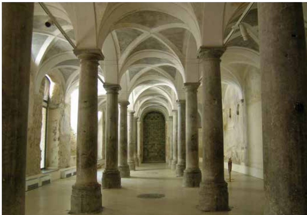
◇ Fig. 16 – Palermo. Palazzo Sambuca, stable with columns made of Billiemi stone (photograph by the author).
