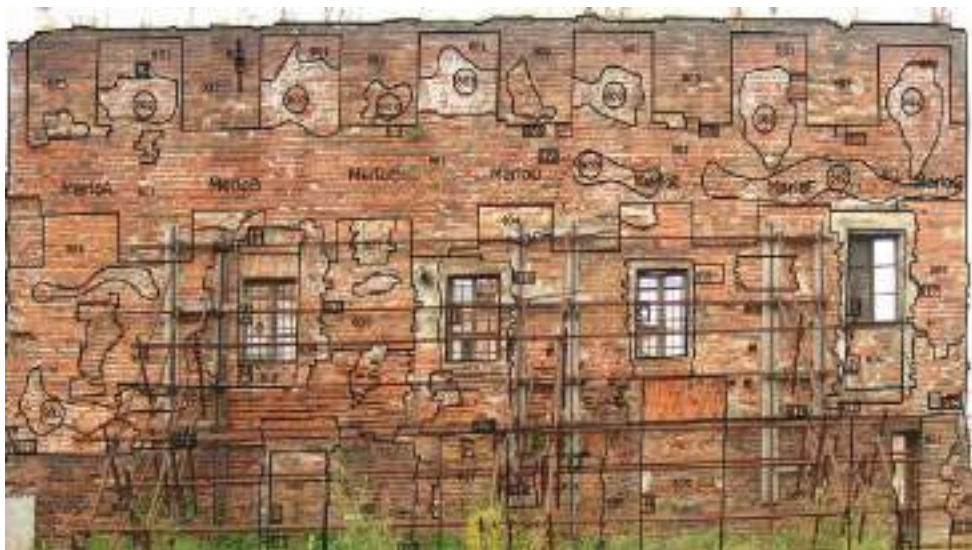
Fig. 7 | Stratigraphic survey of the western facade of the wall (credit: Albani, Gambaro and Mittermair, 2005).
