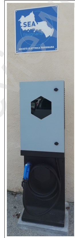
Figure 2. AME V2G charging point, operated by SEA S.p.A. (DSO in Favignana) and installed in Favignana as part of the BLORIN project.
