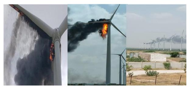
**Figure 3.** Extend of damage due to wind turbine failure during October 2022 at Sapphire Wind Power Plant at Jhimpir.
