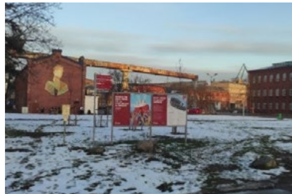
Fig. 8. Directorate building of the shipyard
