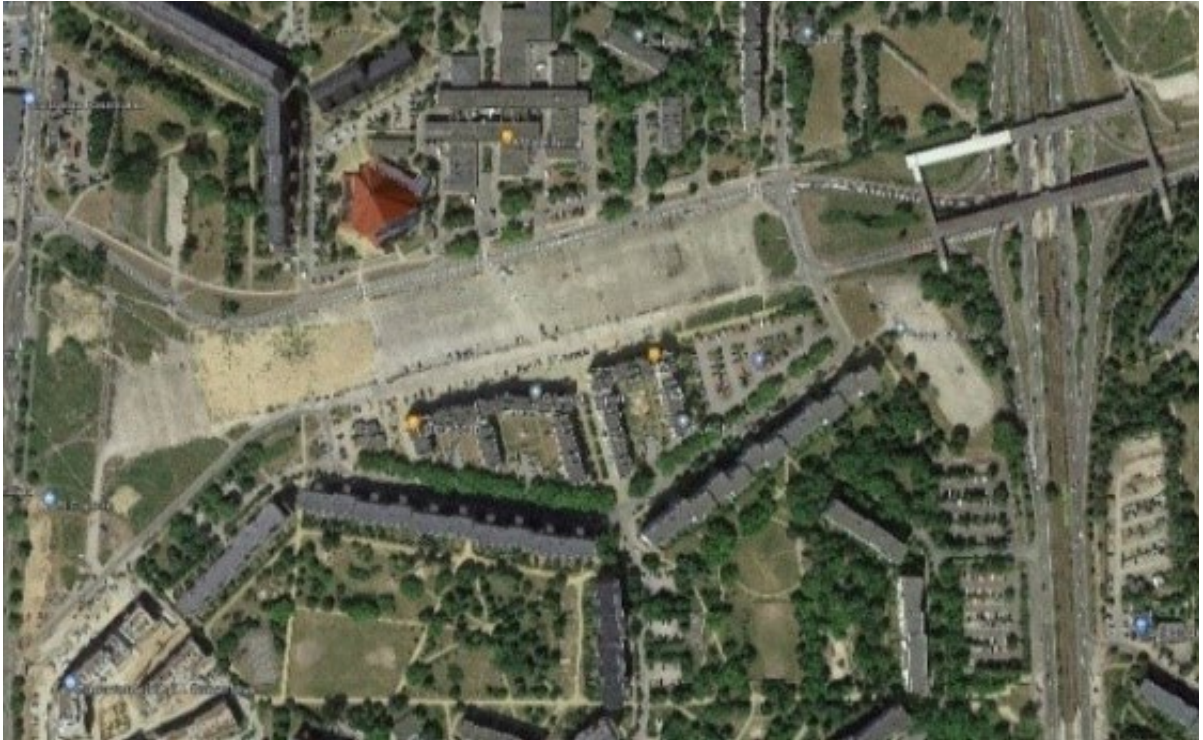
Fig. 2. Existing situation of the runway ,2022
