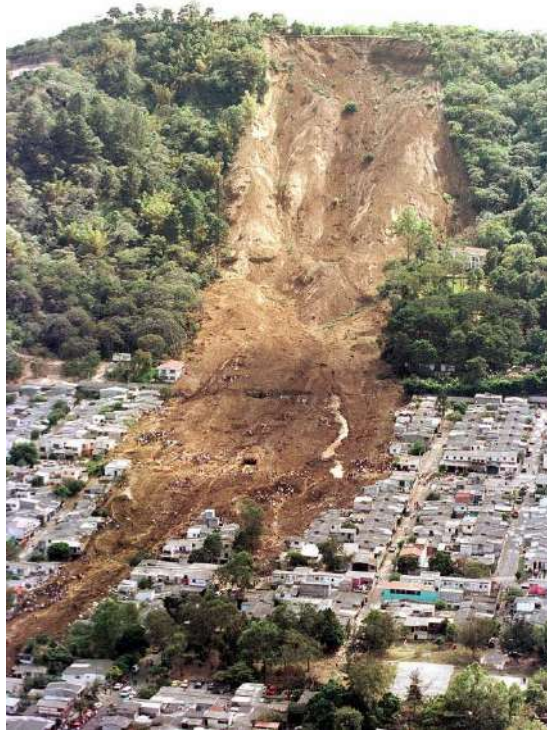
Figure 4.1.1.2: the January 2001 earthquake-induced slide that demolished much of the Las Colinas neighbourhood of Santa Tecla, a suburb of San Salvador (from United States Geological Survey)
