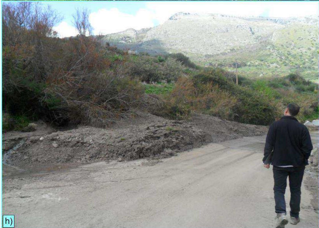
Figure 5.2.3: translational slides; main scarp (g) and landslide accumulation (h) of the 2015 rotational slide affecting the SS643 national road.
