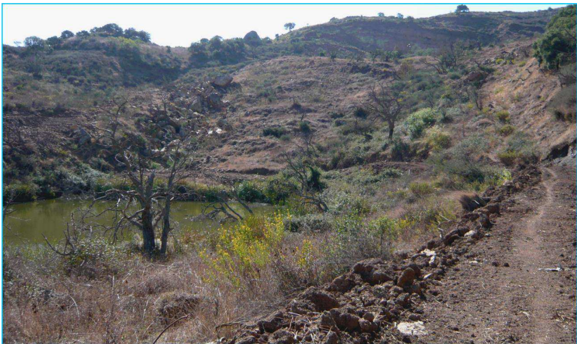
Figure 5.5.2: landslide scarp/head sector of the rotational slide/flow complex landslide in the Suvari area
