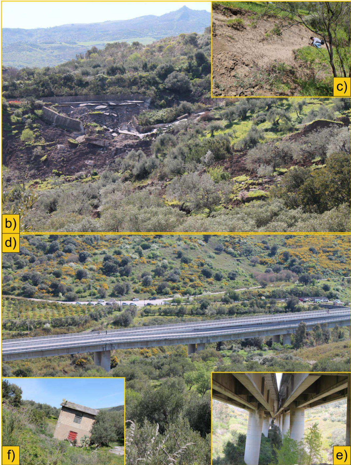
Figure 5.5.2: lateral (b) and main (c) scarps and damaged sectors (d, e, f) at the foot area of the 2015 rotational/flow complex landslide affecting the A19 motorway
