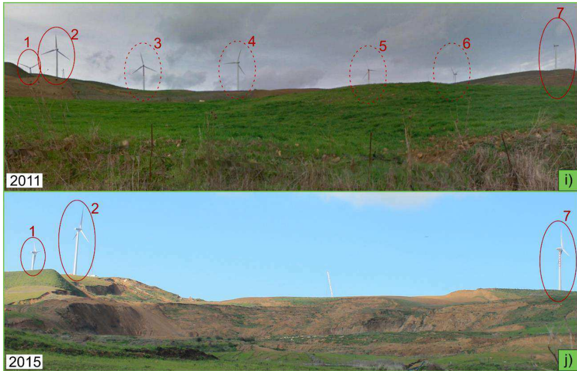
Figure 5.5.4: damage caused to a wind farm (i, before; j, after) in the head zone of the rotational slide affecting the SP53 country road.
