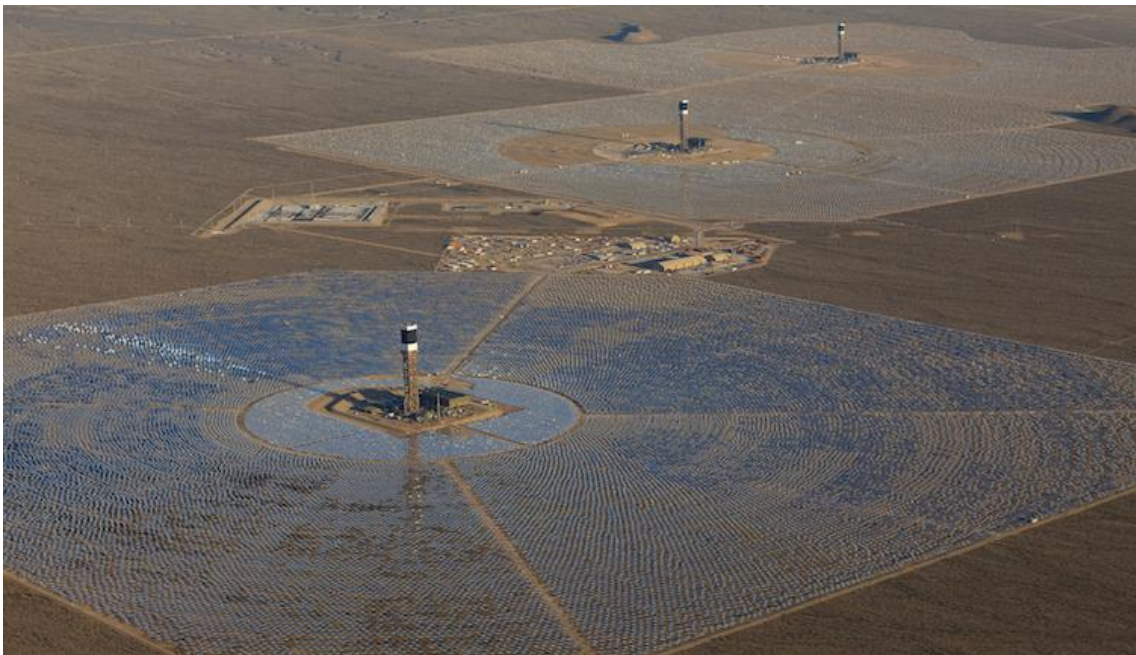
Figure 4. Ivanpah, the largest tower solar CSP plant with a generation capacity of 392-MW located in the Mojave Desert of Southern California (Source: https://www.energy.gov/lpo/ivanpah )
