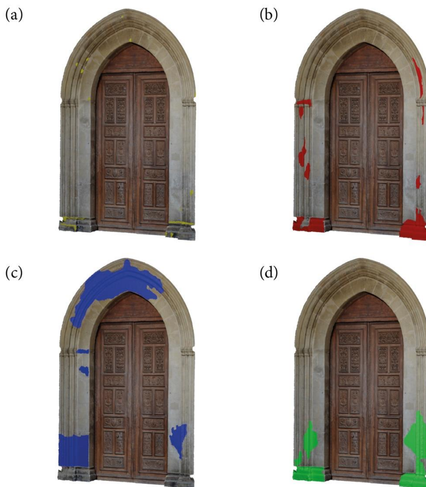
Figure 3. 3D mapping of the four degradation areas: (a) loss of material; (b) erosion; (c) chromatic alteration; (d) black crusts.
