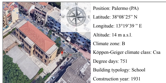
Fig. 1. General characteristics and south-east elevation view of the Rosmini School building.
