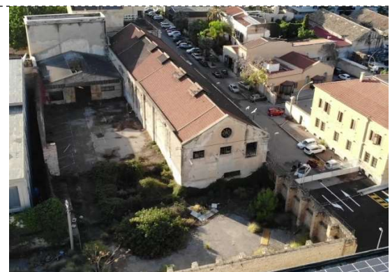
Figure 4. Aerial view of the actual state of the Volta power station.
