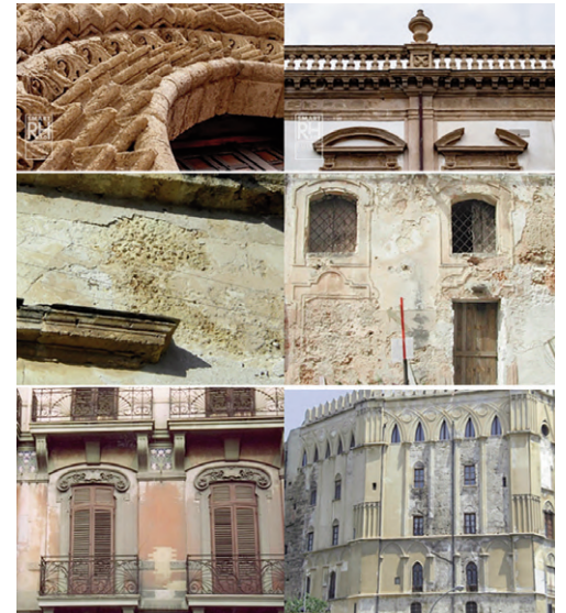
Fig. 10 | Different colours of historical buildings in Palermo: ocre yellow limestone, white plaster or stucco, plaster simulating red bricks, fake stone plasters (credit: F. Renda, 2021; T. Campisi, 2002).
