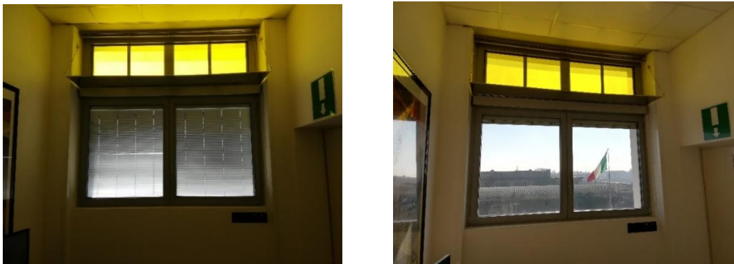
Figure 16 - (a) Shading system in the configuration of the window completely closed – (b) Shading system in the configuration of the window completely opened
