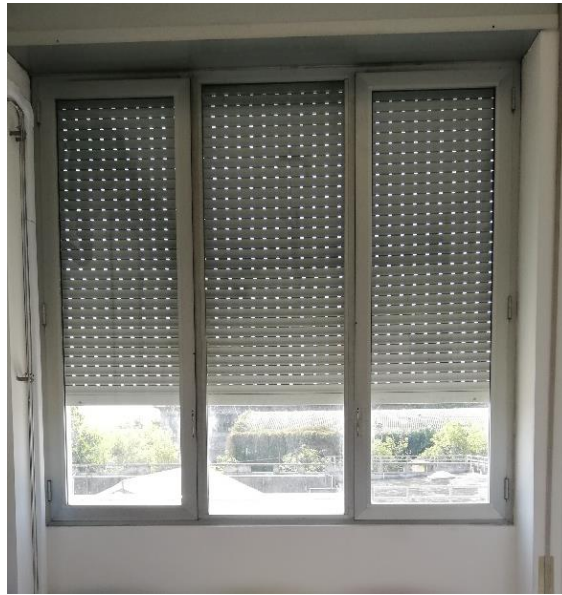
Figure 17 - The traditional window located on first floor
