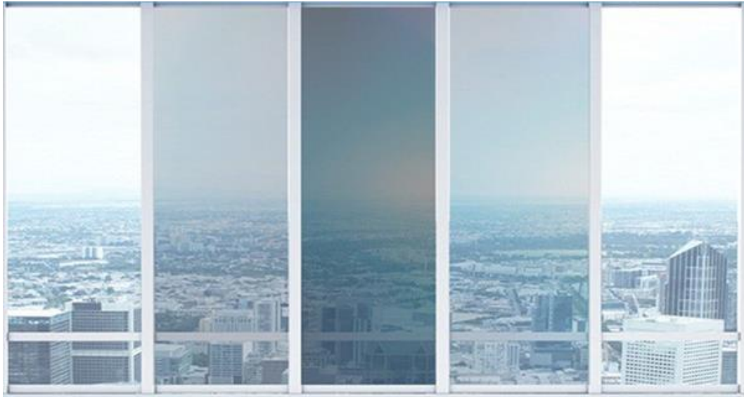
Figure 8 – The visual effect of a photochromic window during different phases
