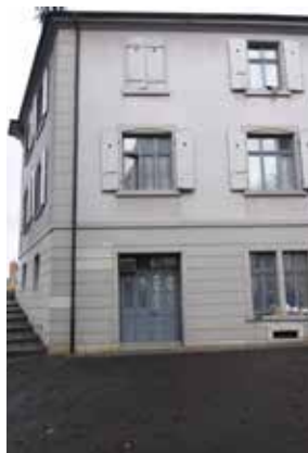
Fig. 1 - Apartment building with Dieter Roth's studio, St. Alban-Rheinweg 52, CH-4052 Basel, Switzerland; Photo: Nathalie Noorlander.
