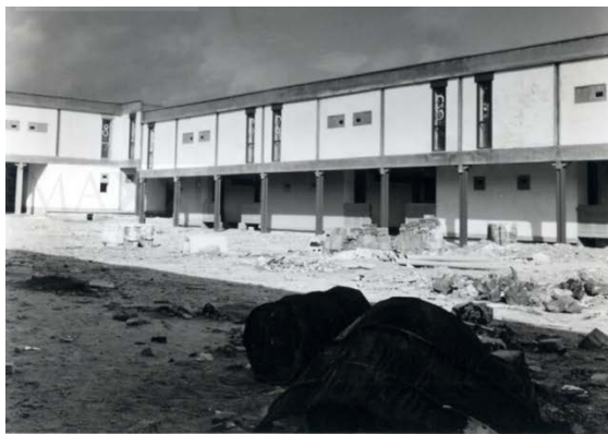
Figure 1. A courtyard during its construction.
