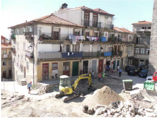
(a) During works, c. 2012.
