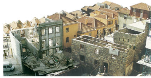
(b) During UPP works, c. 1996.
