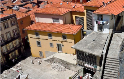
(c) During URP works, c. 2009.
