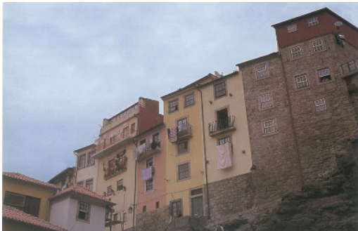
(c) After UPP intervention.
