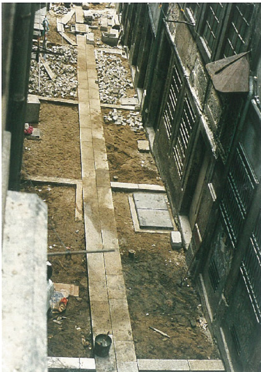
(a) During works, c. 1996.
