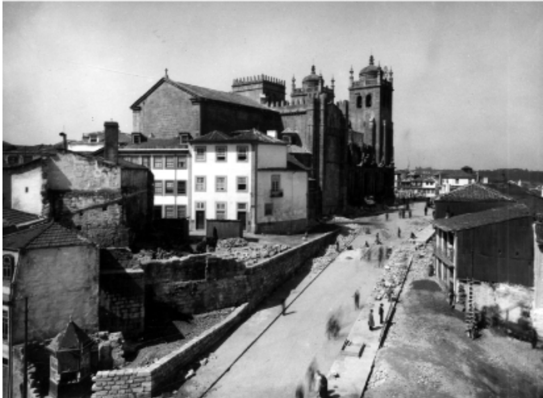
(c) After first demolitions.
