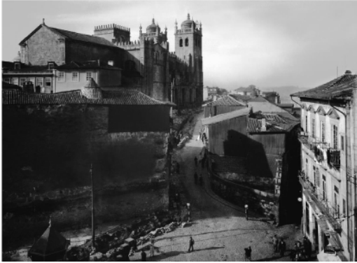
(a) Before demolitions.
