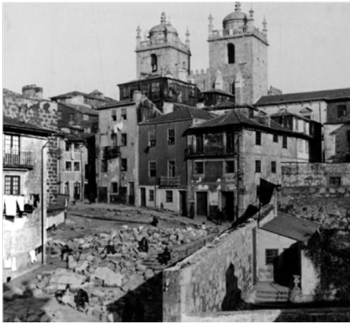
(a) Before demolitions.
