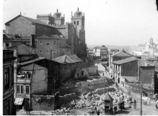
(b) During demolitions 1940s.
