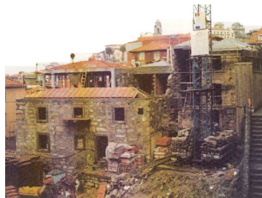
(b) During works, April 1998.
