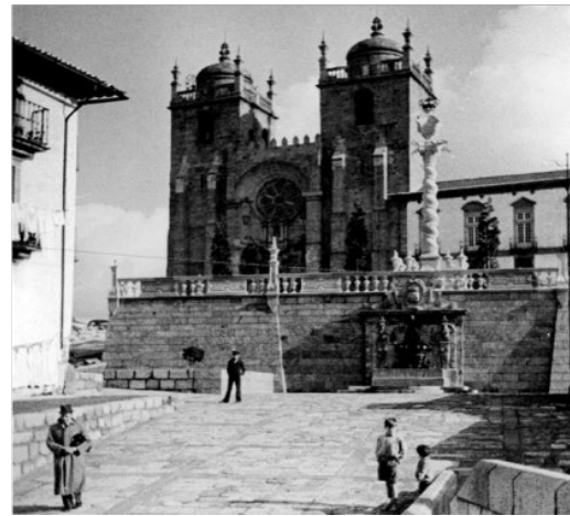
(b) After demolitions.
