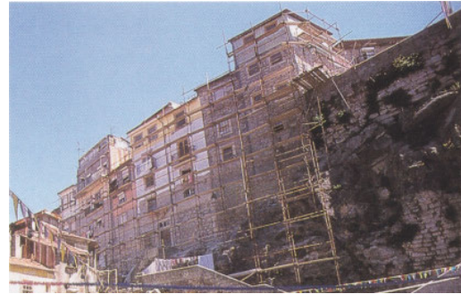
(b) During rehabilitation.
