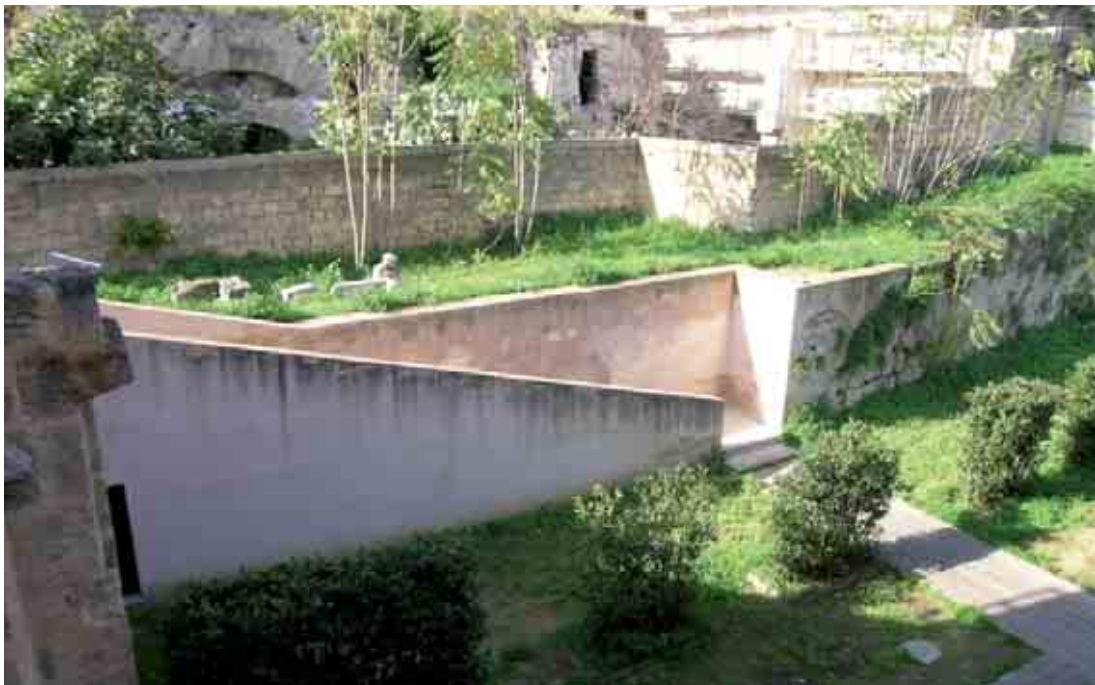
Fig. 11 Palermo, 'Palazzo Belmonte-Riso'. New staircase of access to the palace from the garden
