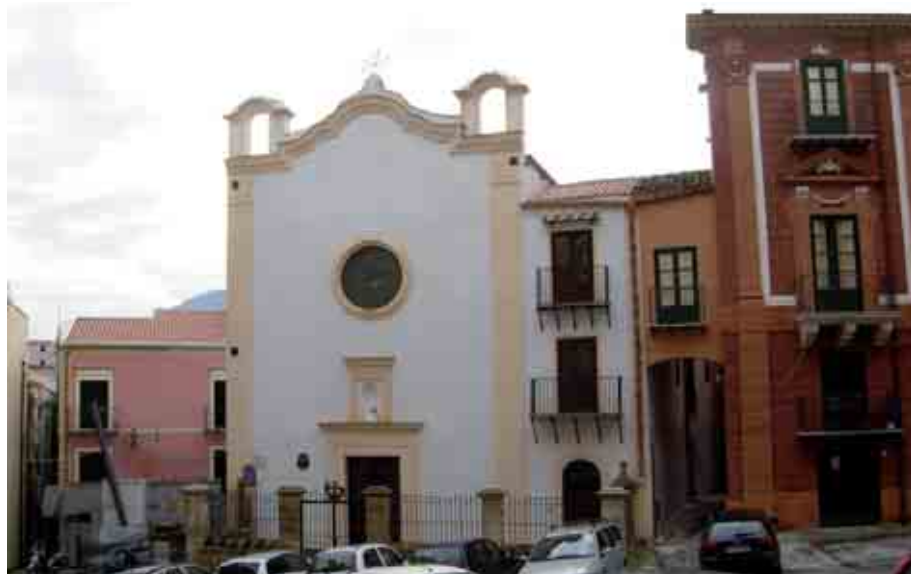
Fig. 6 Palermo, church of 'San Giovanni Decollato', in the district of 'Palazzo Reale'
