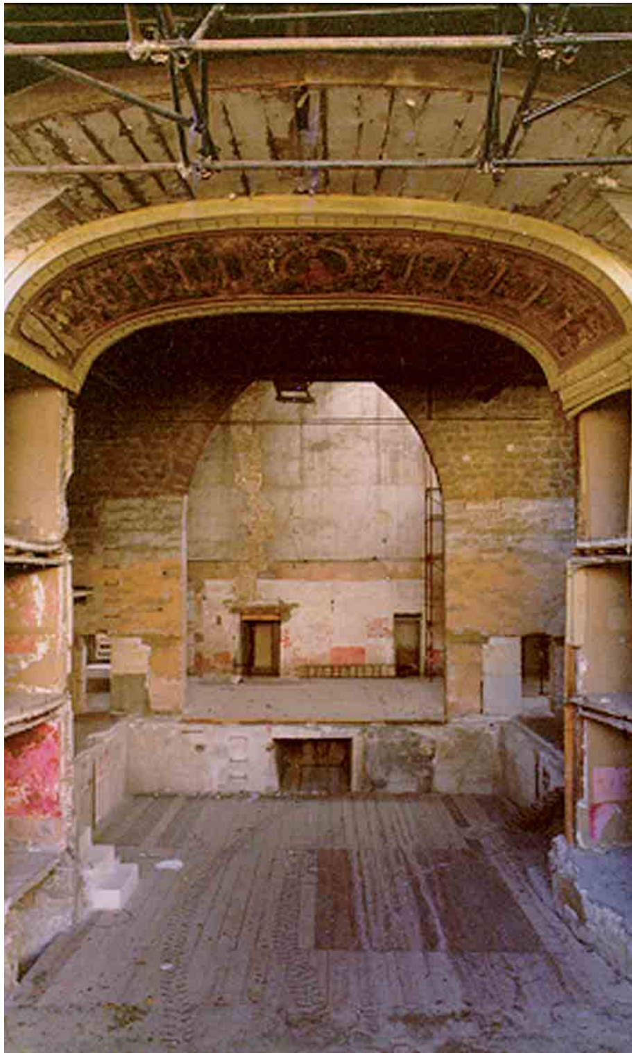
Fig. 20 Palermo, 'Teatro Garibaldi' after the first reinforcing interventions
