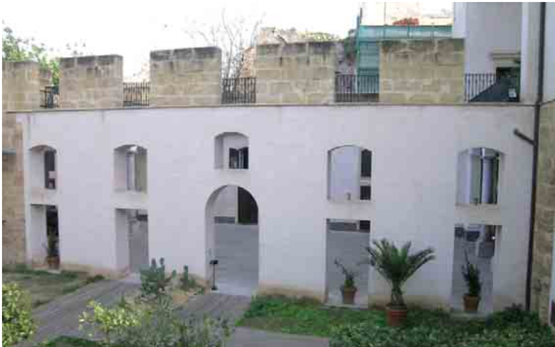
Fig. 10 Palermo, 'Palazzo Belmonte-Riso'. Outside view on the face walls of the courtyard.
