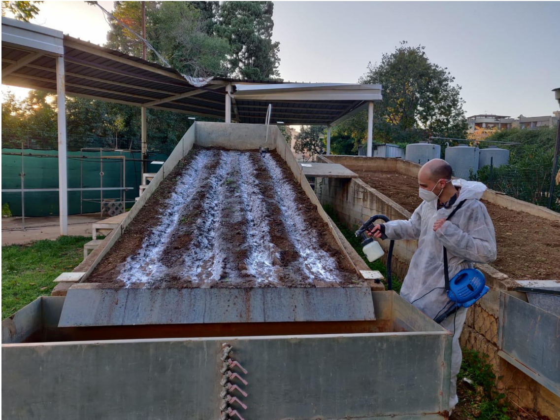
Figure 13. Fixing bed rills with mixture of waterproof vinyl glue and water.
