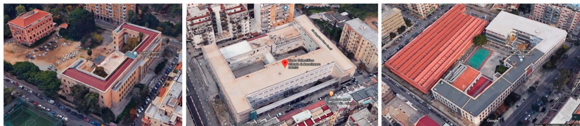
Figure 2. The three school buildings in Palermo.
