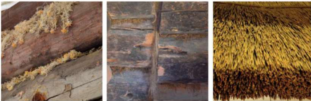
Fig. 3: Dry moss, and flax tow used to ensure thermal insulation between the logs (a,b), straw for the roof coating (c).
