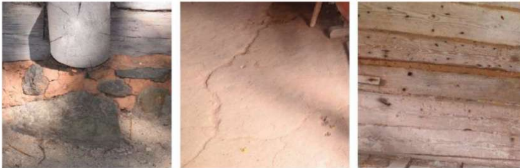
Fig. 2: Clay used for foundation reinforcement, indoor flooring, and to fill the spaces between the wall trunks.
