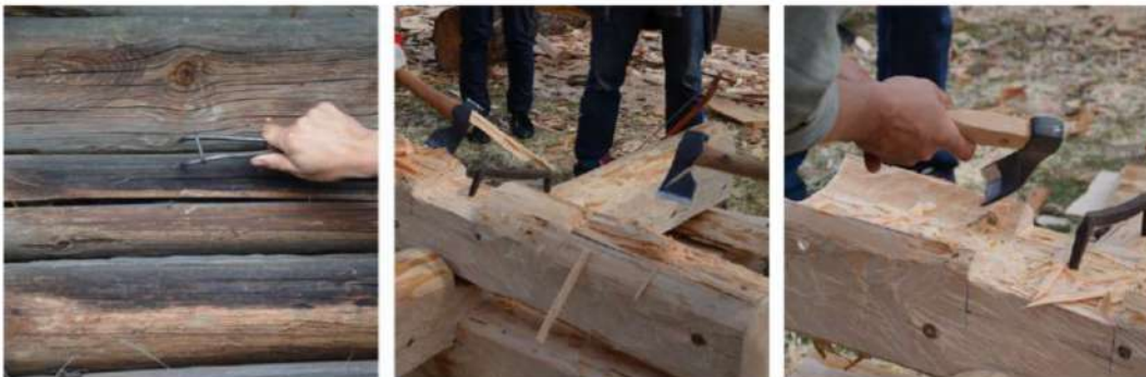
Fig. 5: Preparation of the log grooves.
