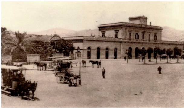
Lolloi station in Palermo, in a historical photo. It was activated in 1891. (C. Pezzillo, La Guilla, foto storiche di Palermo in laguilla.wordpress.com ).
