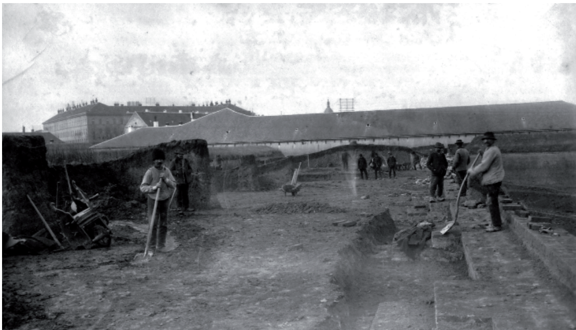
Workers involved in demolition of walls in a picture of the time. (source: Ciprian Glăvan, Defortificarea cetății Timișoara in «Analele Banatului», S.N., Arheologie – Istorie, XXI, 2013, p. 430)
