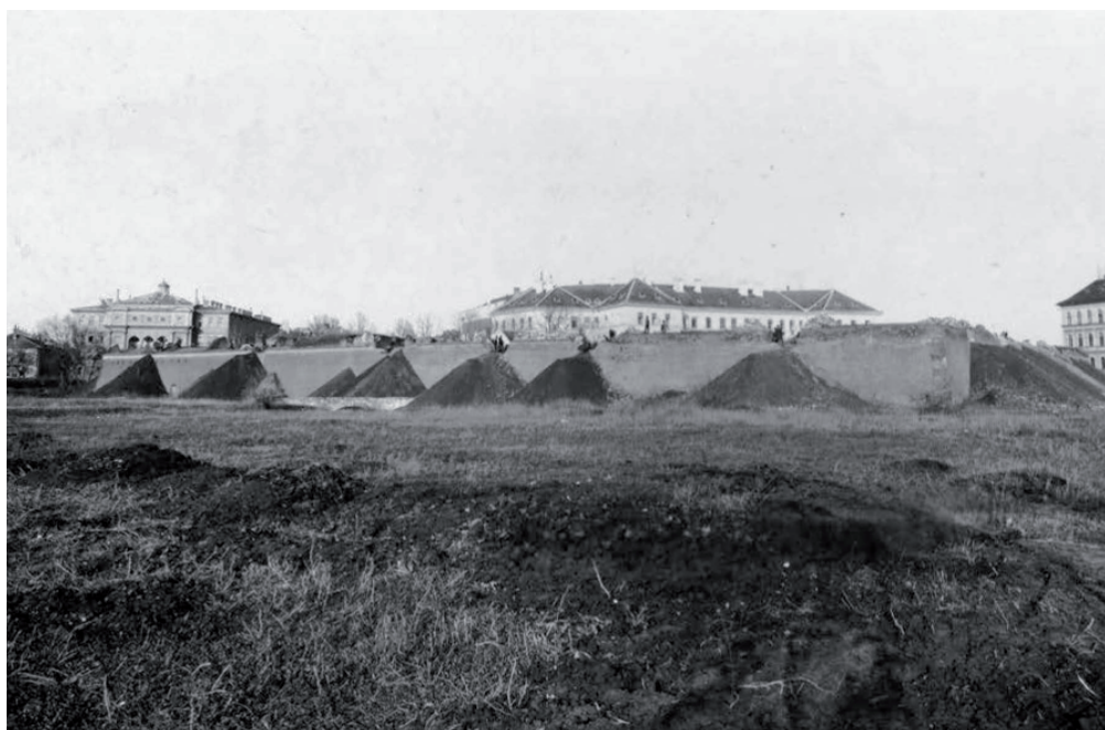
Defortification works near Huniade Castle bastion. (source: Ciprian Glăvan, Defortificarea cetății Timișoara in «Analele Banatului», S.N., Arheologie – Istorie, XXI, 2013, p. 429)
