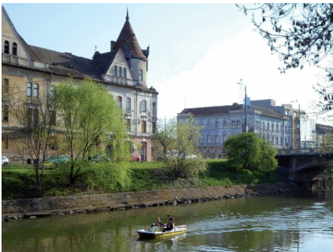
fig.42. Ancora palace in the foreground. In the background the Hotel Royal, Palatul Károly Weisz, in a current photo. (photo by Costica Liciu, 2014).
