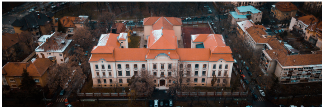
fig.19. Timișoara. College "Constantin Diaconovici Loga" . A block view from which you can read the planimetric system. (www.cdloga.ro, Colegiul Național C. D. Loga, 2017).
