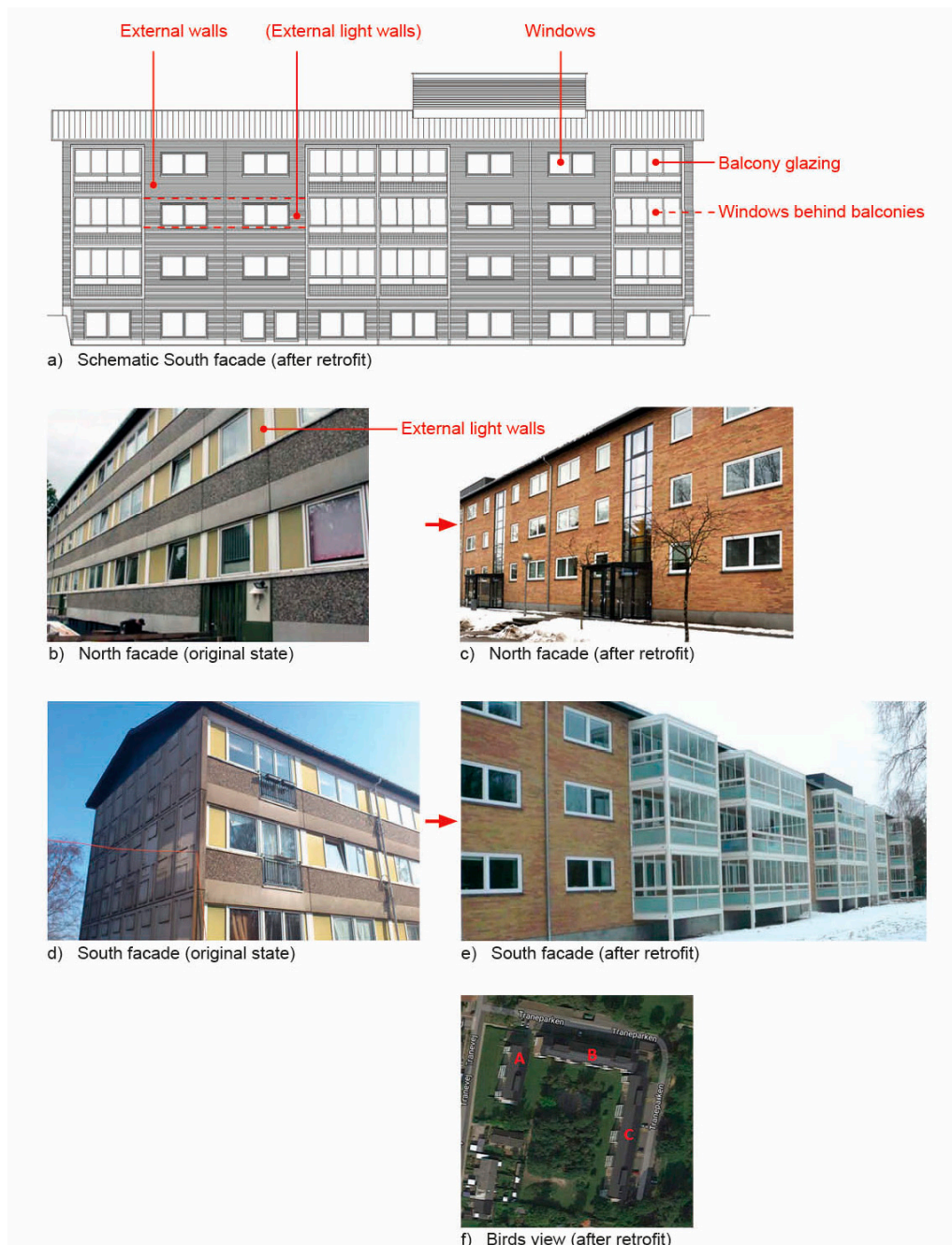
Figure 2. The social housing scheme “Traneparken” before and after the renovation.
