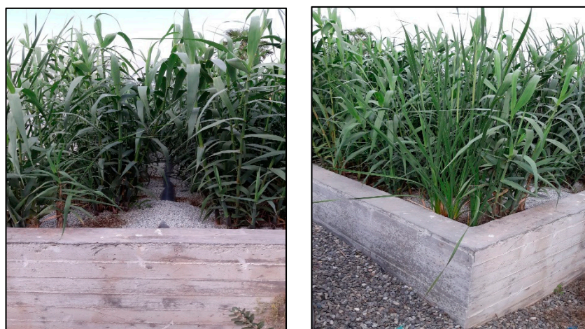
Figure 1. An overview of the vertical subsurface flow system (VSSFs) constructed wetland (CW) at ExpA_1.
