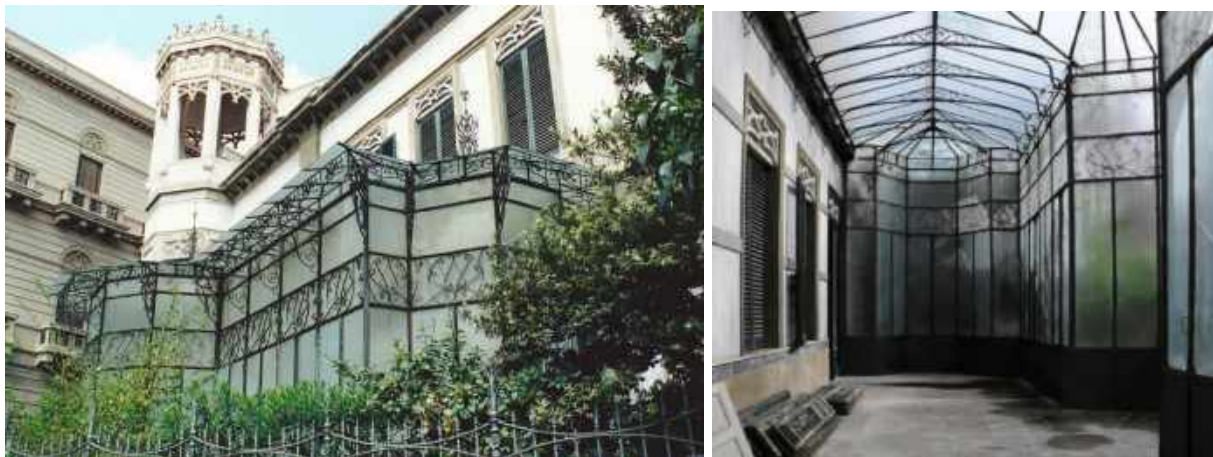
Fig. 7: Exterior and interior view of the winter garden of the Villino Favalaro by E. Basile
