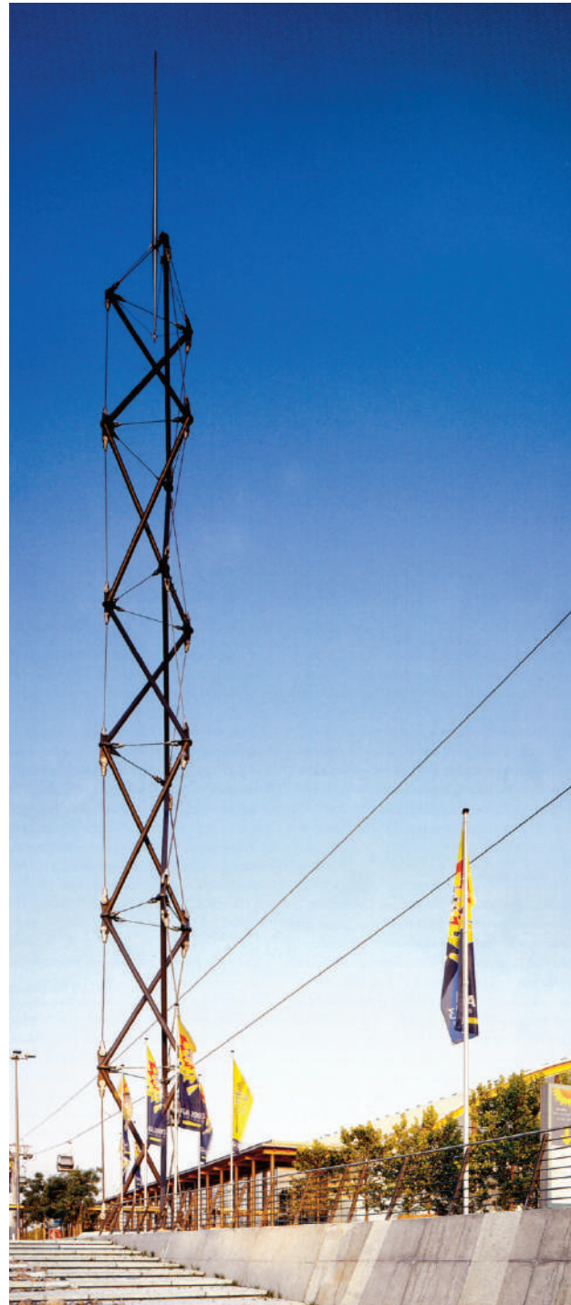
Fig. 5, 6 - Tensegrity T-prism; Gerkan, Marg und Partner (Architect) and Schlaich, Bergermann & Partner (Structural Design), Tensegrity Tower, Rostock, 2003 (H.G. Esch, Hennef-Stadt Blankenberg).
