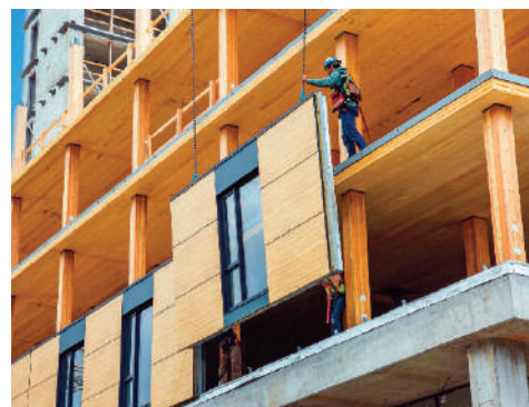
Fig. 4, 5 - Building site as ‘assembly’ place; Prefab housing module, just before to be ‘plugged’.
