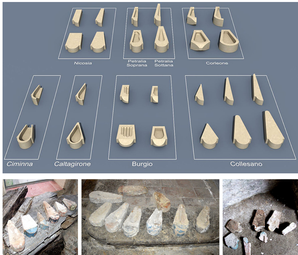
Fig. 2. Sicily, shaped wedges: up, three-dimensional reconstructions of some of the most frequent cases; down, examples of wedge-shaped bricks used in the same spire with different tapering angles.
