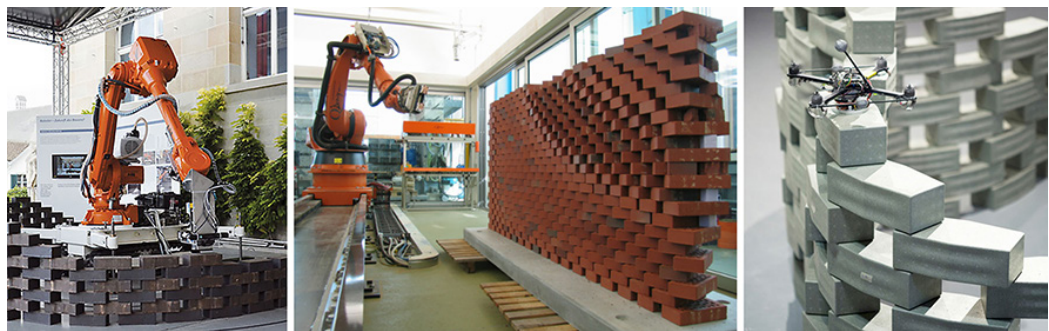
Fig. 6. Construction of masonry walls with robotic arm systems (Gramazio and Kohler from ETH Zürich) or with the use of drones.
