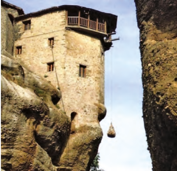
Fig.01 The Greek monasteries of “Metéora”, built on the summits of rock formations average 300 mt in height, offer an archetypal example of mechanical vertical mobility: “before the 1920s ascending the rock columns involved the perilous enterprise of climbing ladders or being hauled up by ropes and nets” ( https://www.britannica.com/topic/Meteora ). Av. at http://www.monastiria.gr/meteores-monastere-de-barlaam/?lang=fr .
