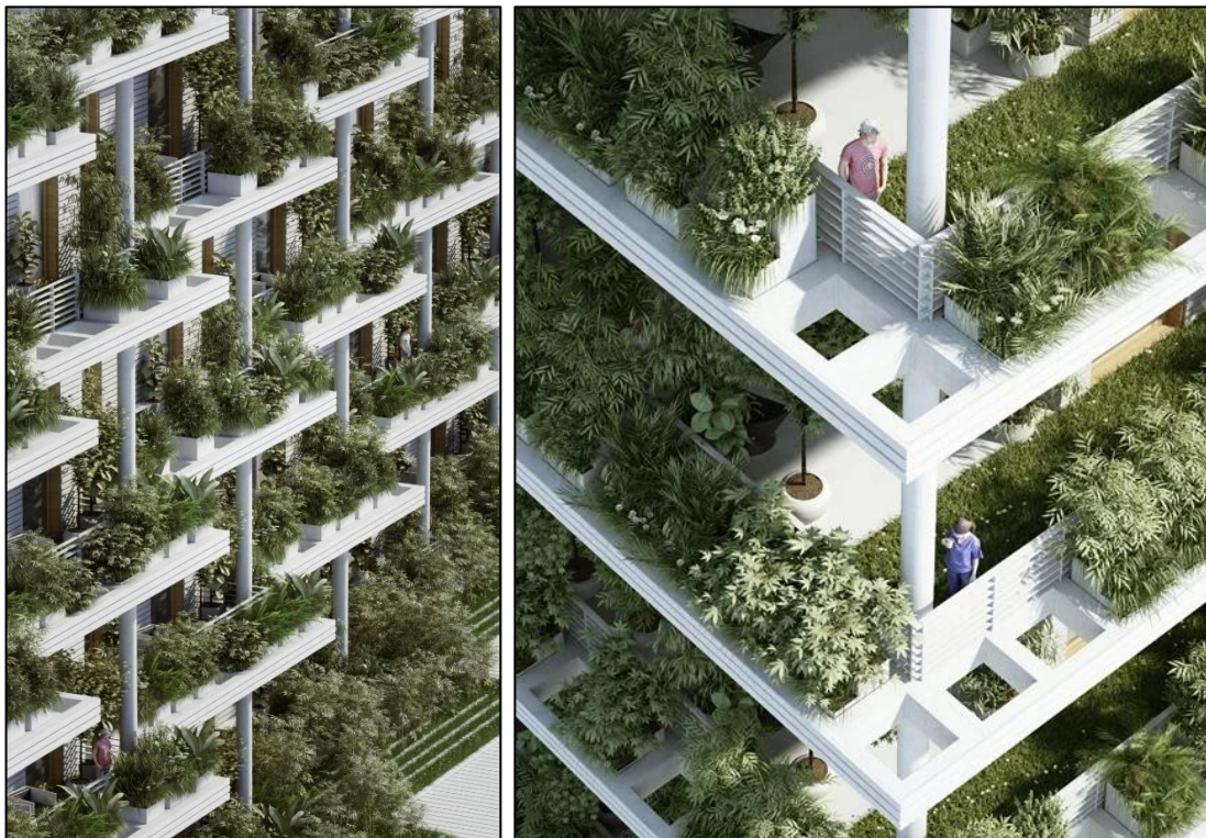
Figure 41 Balcony planters (Designboom, 2016).
