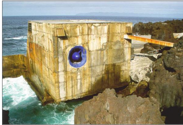
Figure III.11 Back view of the OWC plant installed on the island of Pico (Azores, Portugal) [158] (Elsevier license n. 4707221496823)
