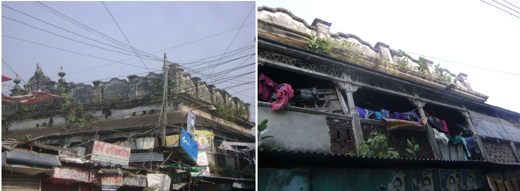
Photograph 5.24: Existing condition of Hindu Hotel
