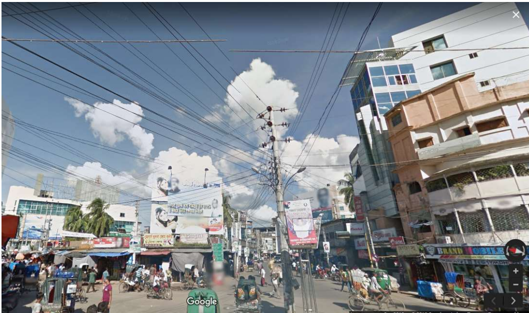
Photograph 5.7: High rise building towards upper jessore road, source: Google map
