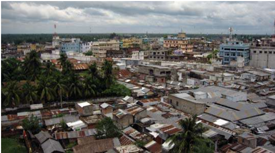
Photograph 5.2: Low structures dominate Boro Bazaar's commercial fabric; Source: Dudek and Evelyne
