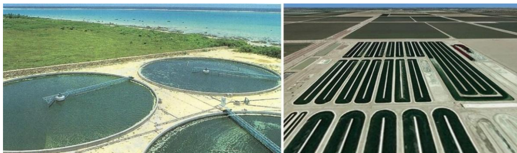
Figure 1.16: Circular and raceway open ponds. A) Chlorella Industries, Japan, circular ponds, each ~500 m 2 , with central pivot mixing B) Cyanotech Co., Hawaii, producing Spirulina (Benemann, 2013).
