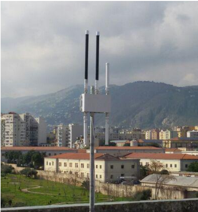
Fig. 7. LoRa Gateway installation.
