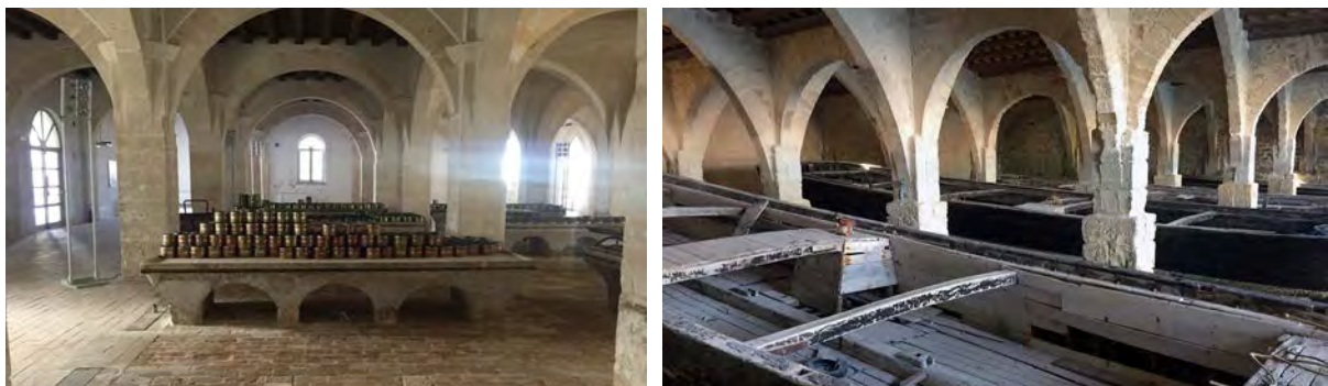
Fig. 6-7: The tonnara building (designed by architect Damiani Almeyda) was built using local calcarenite.
