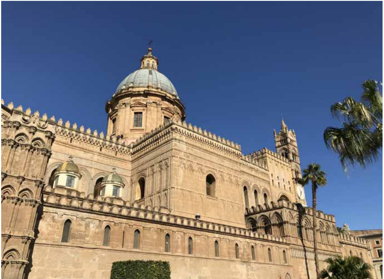
Figure 2 Palermo Cathedral: southern façade (photo: author)
