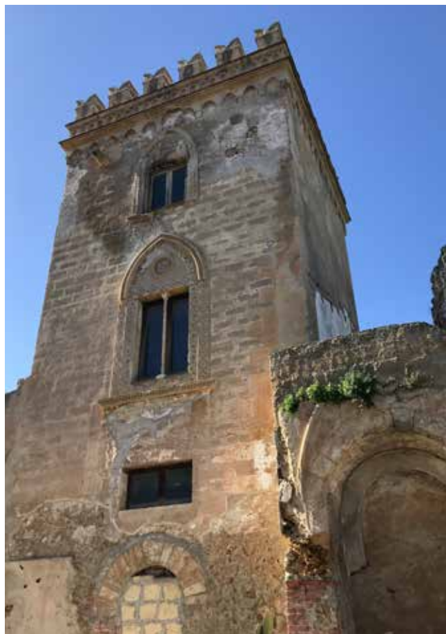
Figure 7 The so-called ‘Milinciana’ tower at Boccadifalco, Palermo, designed by Gaetano Bernasconi, 1810–15 (photo: author)
