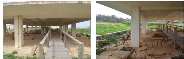
Figure 3. Wooden walkways on the Roman Domus .
