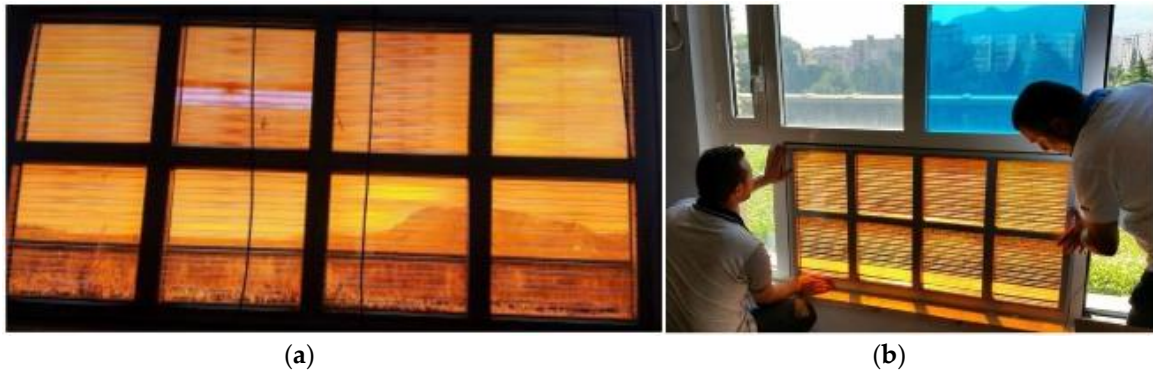
Figure 7. Set-up of the three PV vertical structures. DSSC PV wall system, made by Daunia solar cell: (a) assembly of 8 modules; (b) photograph taken during installation on the window.
