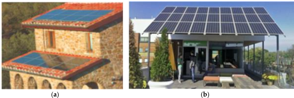
Figure 1. Some examples of building-integrated photovoltaic (BIPV) systems on buildings: (a) country house; (b) modern building.
