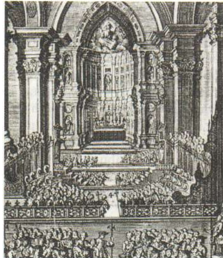
Fig. 8. Engraving depicting the interior of the Palermo cathedral, detail of the Tribune reconfiguration by Antonello Gagini (from SCHIAVO, D., Descrizione della solenne acclamazione... , Palermo 1760).
