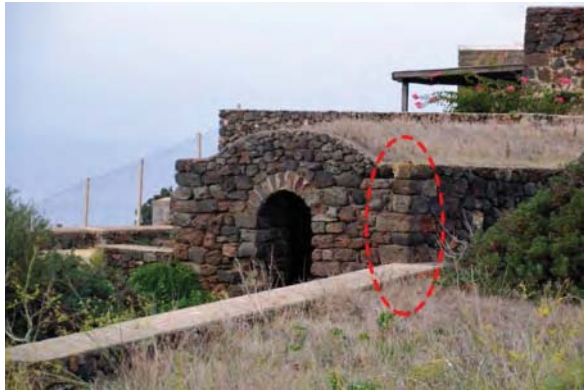
Fig. 4: Particular of the ashlar of a corner.
