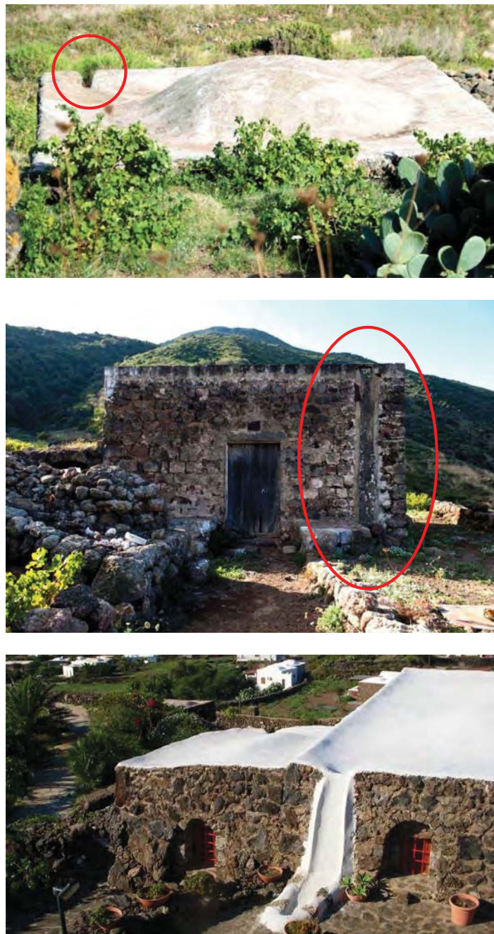
Fig. 9: White superficial lime coating and different disposal systems. Top and centre: a hole in the edge is used to collect water in a wall dig; bottom: a ramp.
