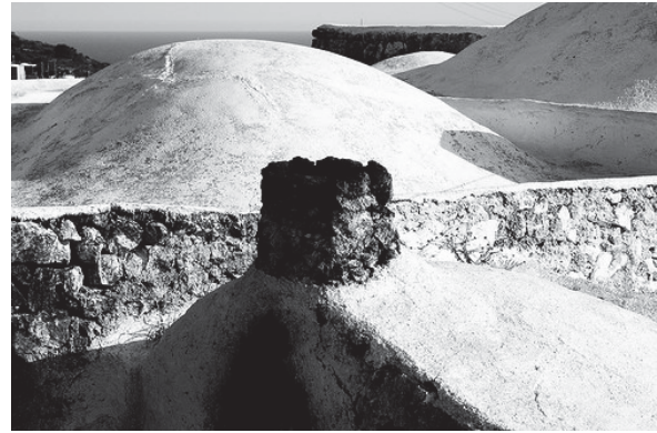
Fig. 7: Typical finishing made of lime mortar.
