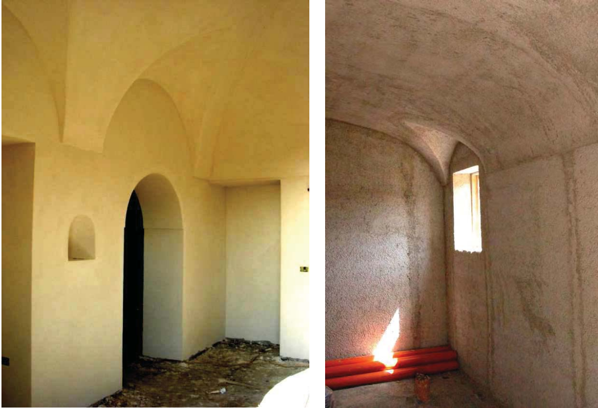
Fig. 13: Cloister vaults equipped with lunettes used to open doors and windows into the walls (figure 13).
