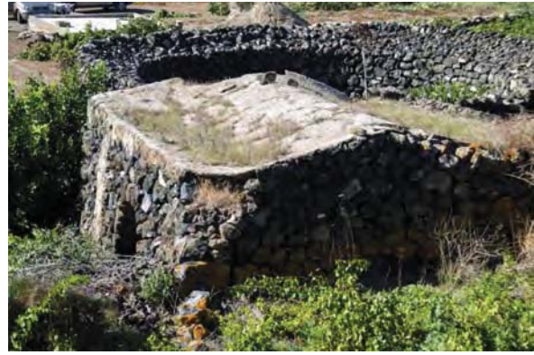
Fig. 6: The oldest typological system of roofing is the real barrel stone vault.
