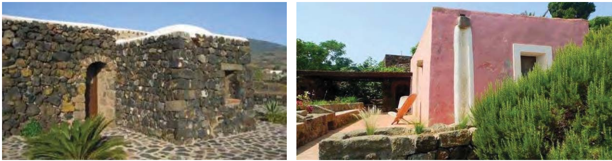
Fig. 10: Traditional external finishing: left – bare masonry stone; right – natural hydraulic lime plaster.
