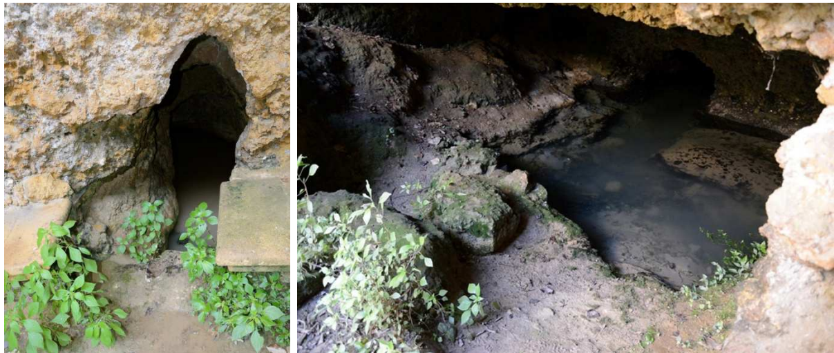
Fig. 9: On the left: passage of access to the qanāt of the Scibene to which comes the water of the canal, now covered, which crosses part of the floor of the chamber. On the right: the collection basin into which the waters captured by the Scibene source and those of the waterfall generated by the Gabriele source flow; ph Carmelo Bustinto.
