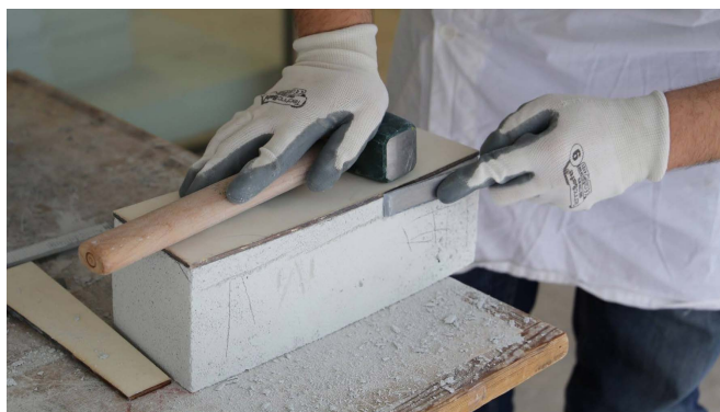
Figures 24, 25. Control of compliance of carved stone, respecting a “modano” model and realization of wooden centering, positioning the dry-carved ashlar to verify the exact matching of surfaces. (©labstereounipa).
