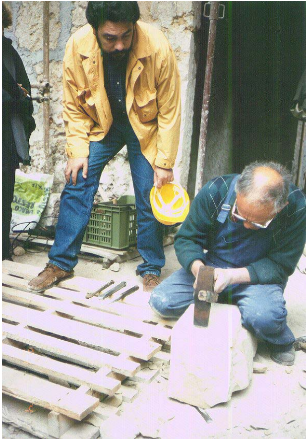
Figures 26, 27. A stonemason shaping the arches ashlar or that supporting the vaults at S. Anna la Misericordia convent.
