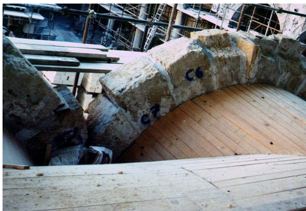
Figures 12, 13. Construction of stony vaults on the realized wooden supporting structure.
