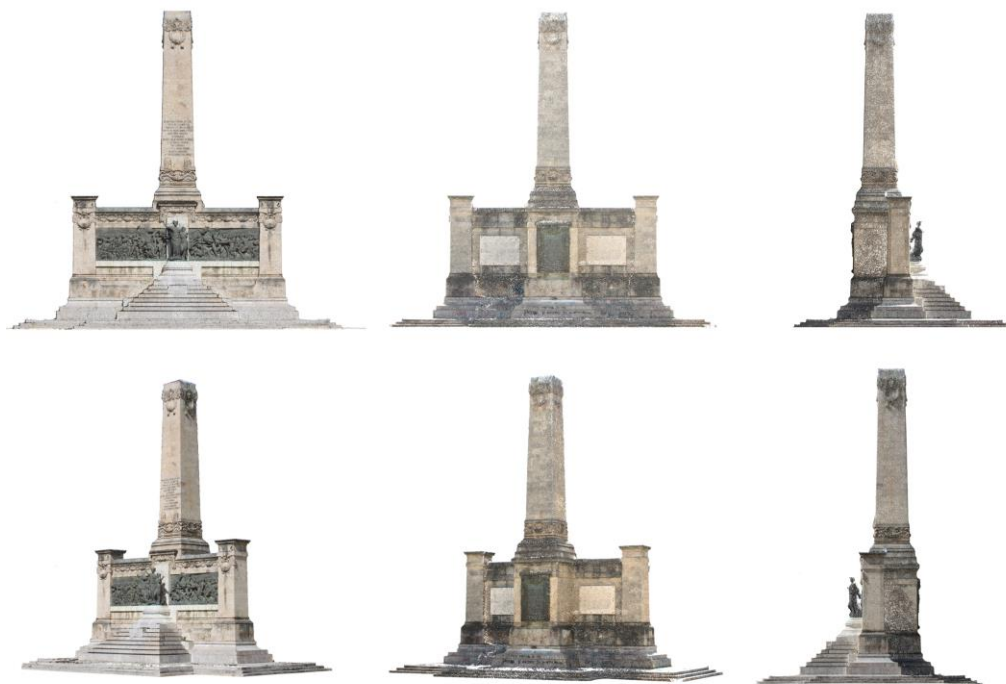
Figure 10. Survey Structure from Motion (by Vincenza Garofalo)
