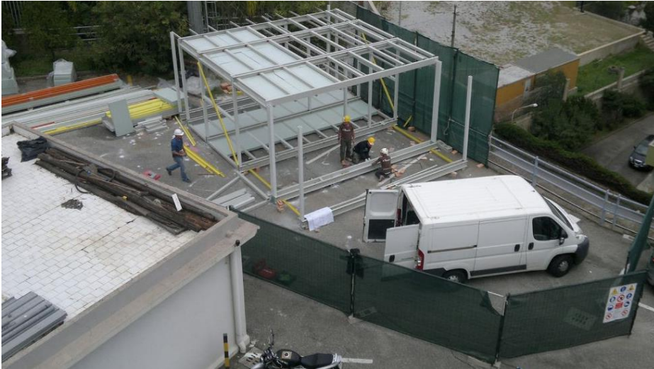
Fig. 4.8 - The case study during the construction stage.
