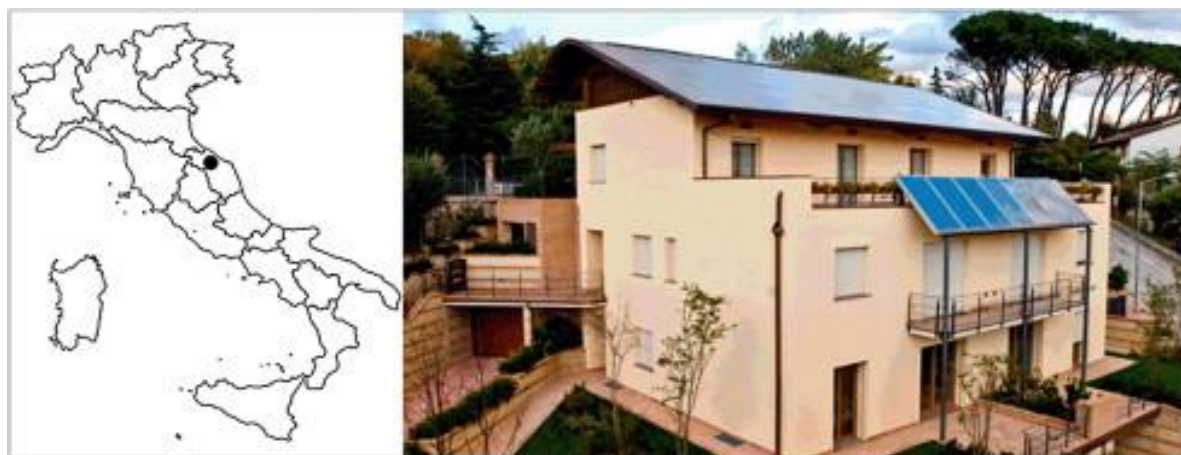
Figure 18. The LH south façade.
