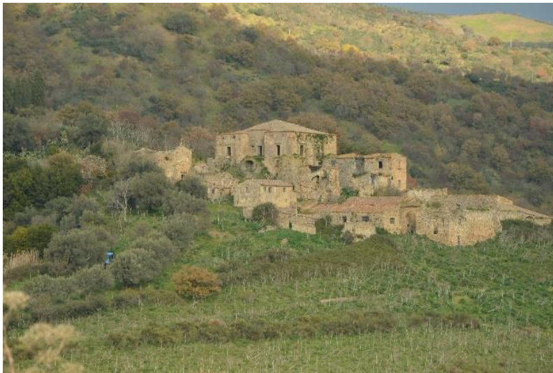
Fig. 2: View of the masseria from the access road
