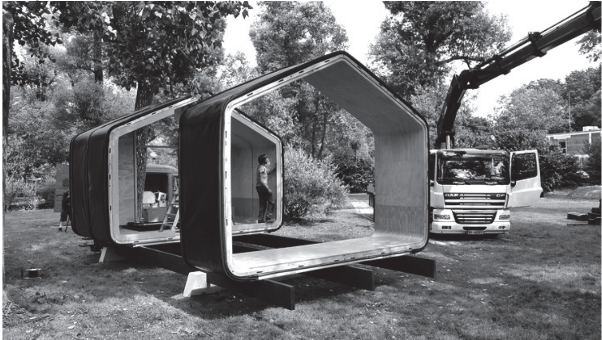
Fig.5: Wikkellhouse (2017), Developed by the Dutch Company Fiction Factory, Is Made Out of Cardboard, Modular and Highly Customisable, Built to Last Between 50 and 100 Years.
