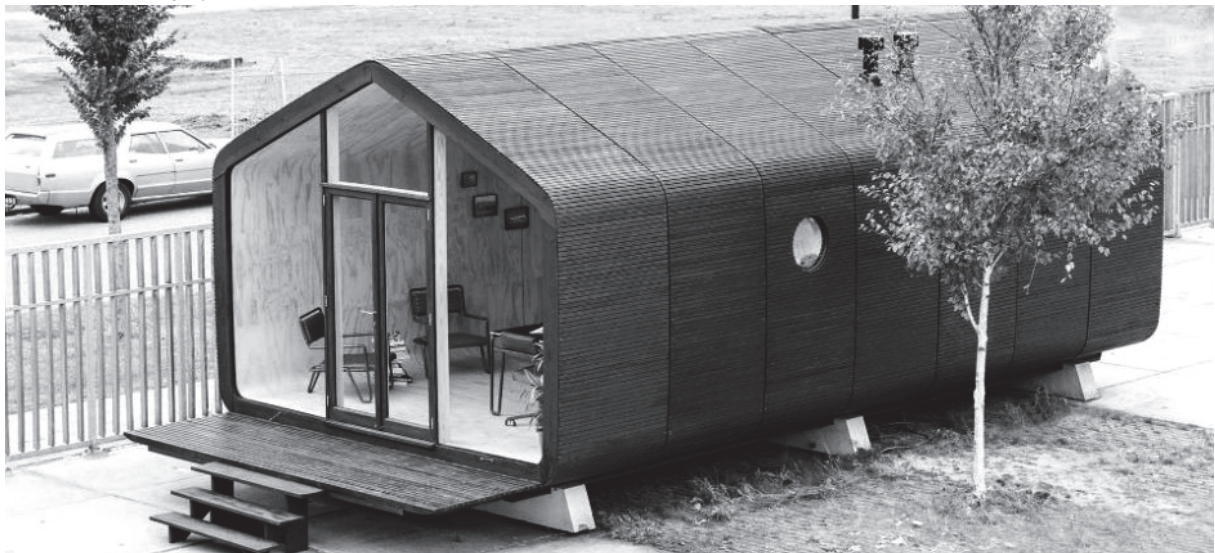
Fig.5: Wikkellhouse (2017), Developed by the Dutch Company Fiction Factory, Is Made Out of Cardboard, Modular and Highly Customisable, Built to Last Between 50 and 100 Years.
