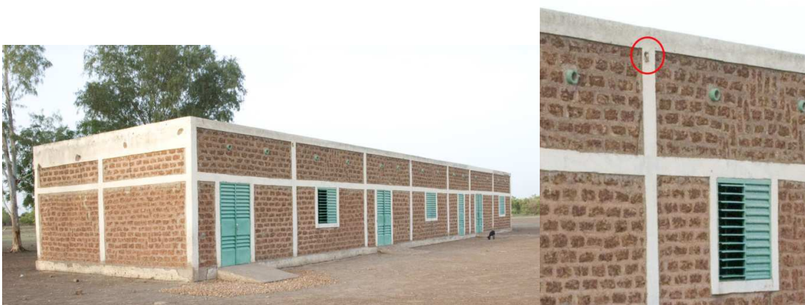
Figure 25. School in Torobà Village
